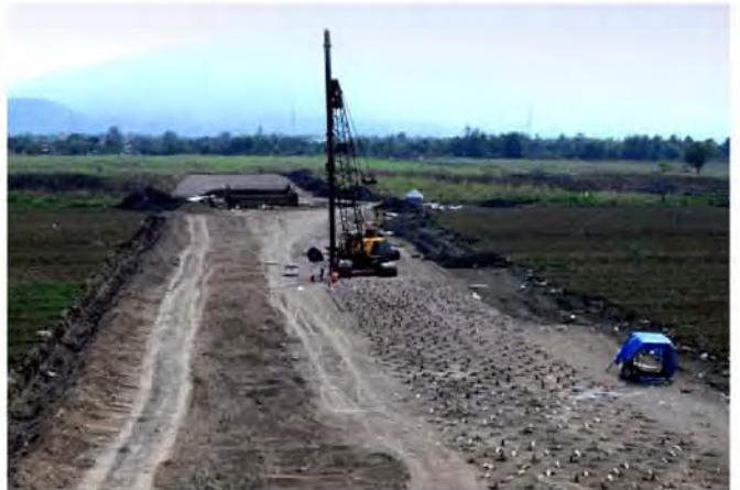
Porong Road Relocation - Package I, East Java, 2009
