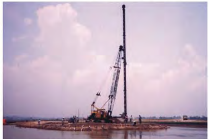
Kaliwungu Road Trial Embankment, Central Java, 2001
