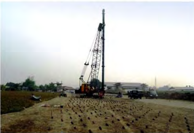
Porong Road Relocation - Package IV, East Java, 2009
