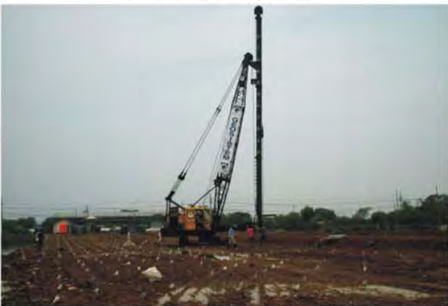
Tanjung Perak Port Access Road, East Java, 2008
