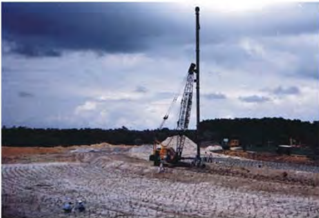
Manggar Dam Improvement, East Kalimantan, 1999
