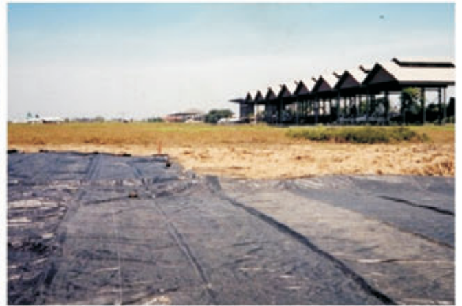
Juanda Airport, PT. Hutan Alam, Sidoarjo, East Java, 1999 (scope of works : geotextile)
