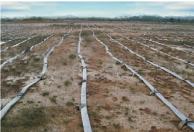
Samarinda Baru Airport, PT. Istaka Karya(Persero), Samarinda, East Kalimantan, 2008 (scope of works : vertical wick drain, horizontal strip drain, geotechnical instrument)
