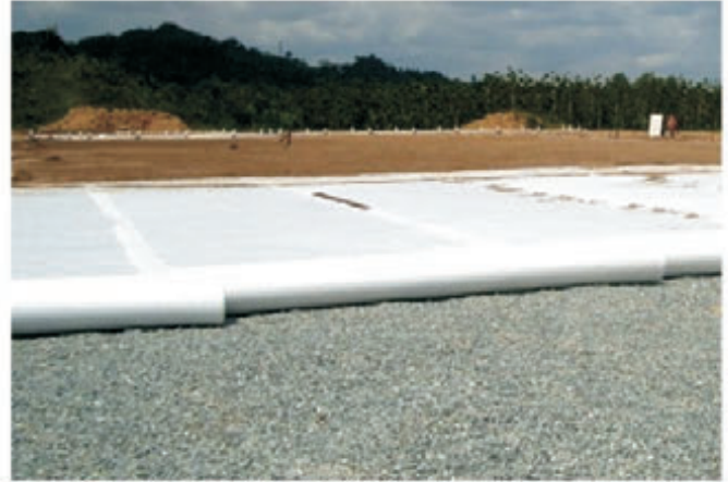
Palaran Main Stadium, PT. Adhi Karya (Persero), Samarinda, East Kalimantan, 2005 (scope of works : geotextile, vertical wick drain, horizontal wick drain)
