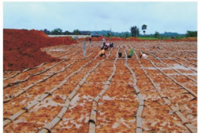
Palaran Main Stadium, PT. Adhi Karya (Persero), Samarinda, East Kalimantan, 2005 (scope of works : geotextile, vertical wick drain, horizontal wick drain)
