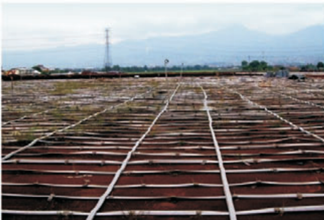
Gedebage Main Stadium, PT. Adhi Karya (Persero) Tbk., Bandung, West Java, 2010 (scope of works : geotextile, vertical wick drain, horizontal wick drain, geotechnical instrument)
