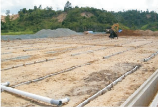
Palaran Main Stadium, PT. Adhi Karya (Persero), Samarinda, East Kalimantan, 2005 (scope of works : geotextile, vertical wick drain, horizontal wick drain)
