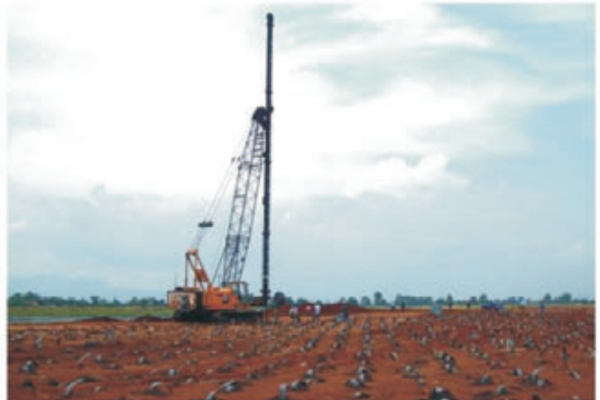
Bung Tomo Main Stadium, PT. Adhi - Rekon JO, Surabaya, East Java, 2008 (scope of works : vertical wick drain, horizontal wick drain, geotechnical instrument)
