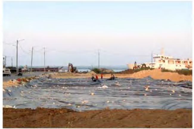
Gresik Container Yard, East Java, 2007
