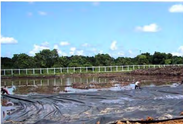
Malinau Airport, East Kalimantan, 2003
