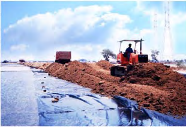
Benowo Sanitary Landfill Access Road, East Java, 1997
